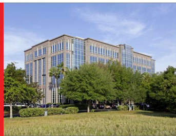
Primera Tower I 610 Crescent Executive Ct Lake Mary, FL
